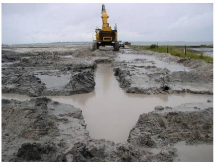
Figure 5. Excavating the trench supported by bentonite slurry
