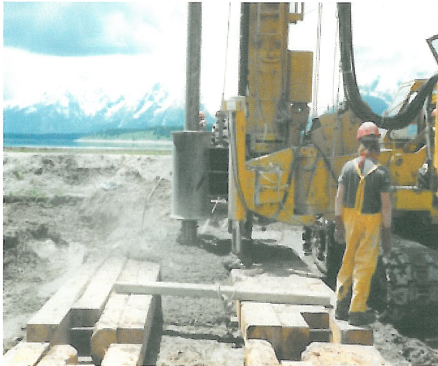
Figure 5. Soil Mixing in Progress
