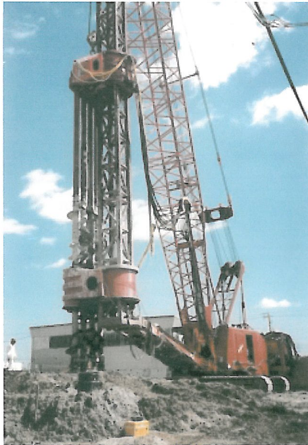
Figure 1. Deep Soil Mixing Drill Rig
