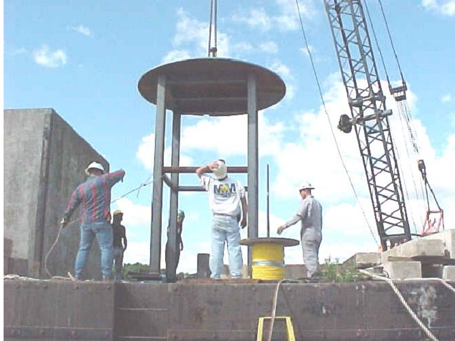
Figure 4. Placing the steel “stool” in the river shaft in preparation for the tremie seal
