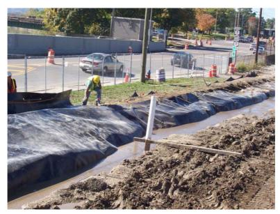
Figure 5 – Placement of HDPE Barrier
