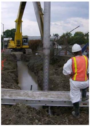
Figure 3 – Jet Grouting
