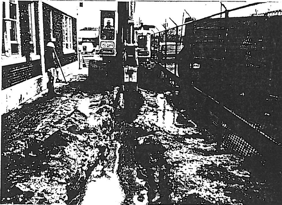
FIGURE 4 - CB WORK IN AREA OF TIGHT ACCESS
