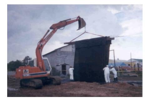
Figure 3. Installation of Geomembrane Panel
