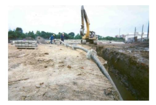
Figure 5. View of Pipe Installation in Bio-Polymer Trench
