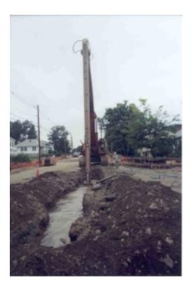
Figure 7. View of Slurry Trench Installation
