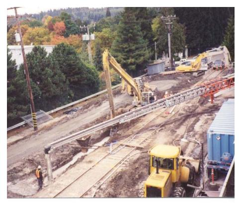
Figure 7: Placing Iron blend In PRB panel in tight site
