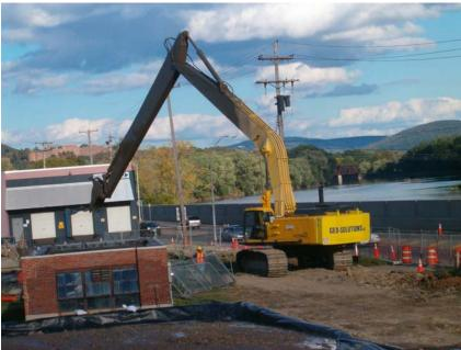
Figure 3: Excavating the Bio Polymer Drain using an extended-reach excavator
