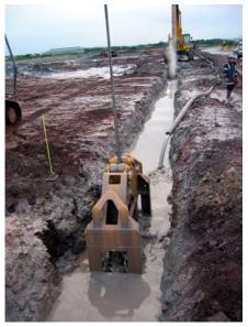
Fig. 1 - Trench excavation for SB wall
