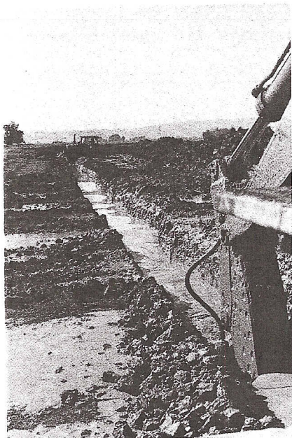
Figure 1: Typical SB Slurry Cut- Off Wall Under Construction
