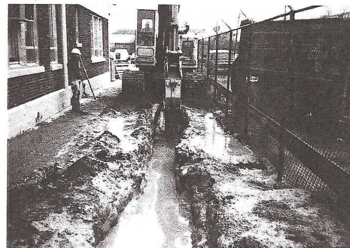
Figure 2: Installing a CB Wall in Tight Quarters
